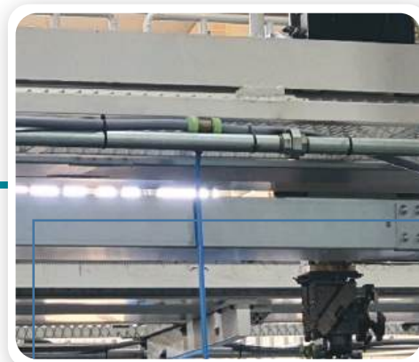
05 Image of a heterogeneous faucet connecting from the PB (Main-Pipe) to the equipment connected to the urethane hose (12A)
